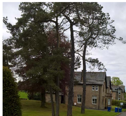
General view within conservation area
