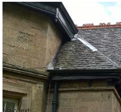
Overlaid zinc flashing over original lead
