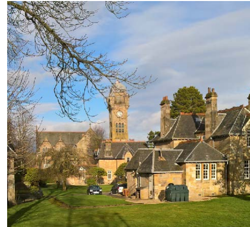
General view towards Mount Zion Church
