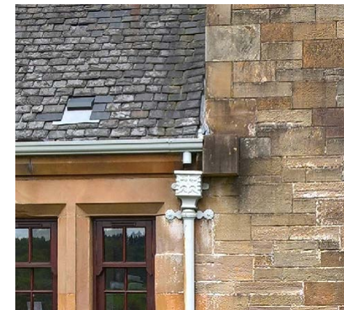
Original cast iron fittings at Glenfarg
