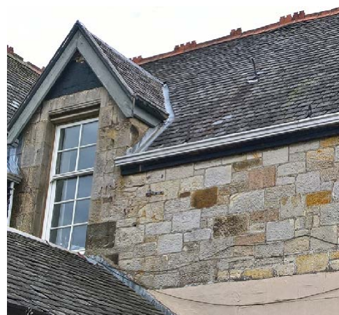
Replacement guttering in aluminium
